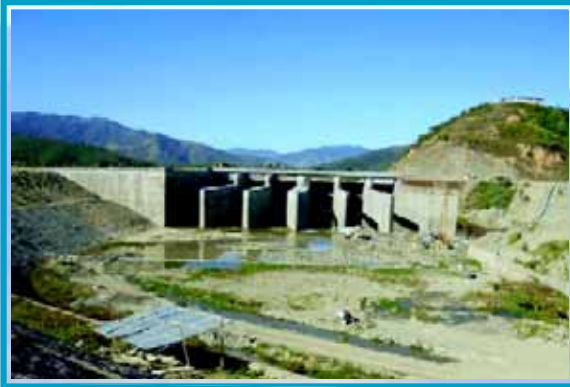
Dolaithabi Barrage, Manipur
