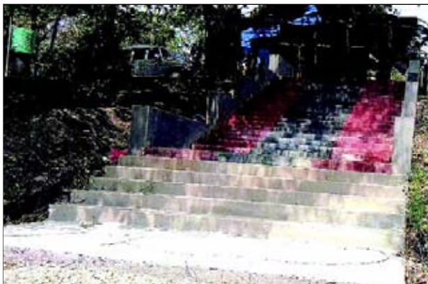
Construction of Pond Ghat at Paschim Medinapur
