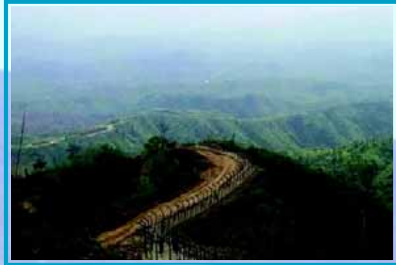
Fencing Work at Indo Bangla Border
