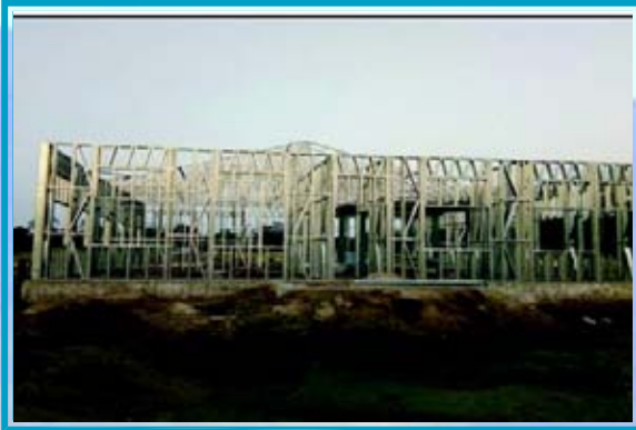
PEB at Solalgaon, Lakhimpur
